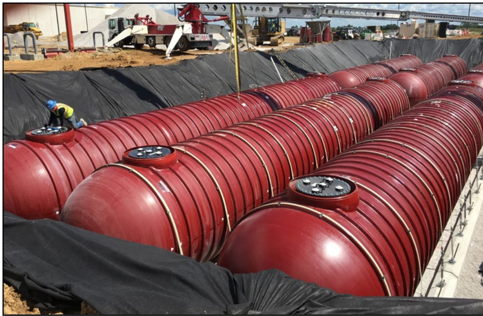
Photo 13 Underground Storage Tank Installation
