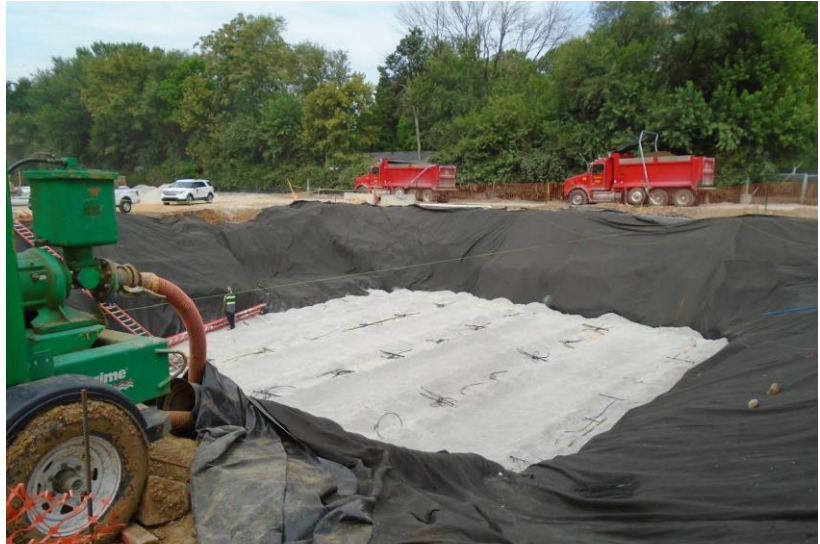
Photo 18: Tank pit area being prepared for installment of USTs. Photo by Rob Staley, Field Office Branch
