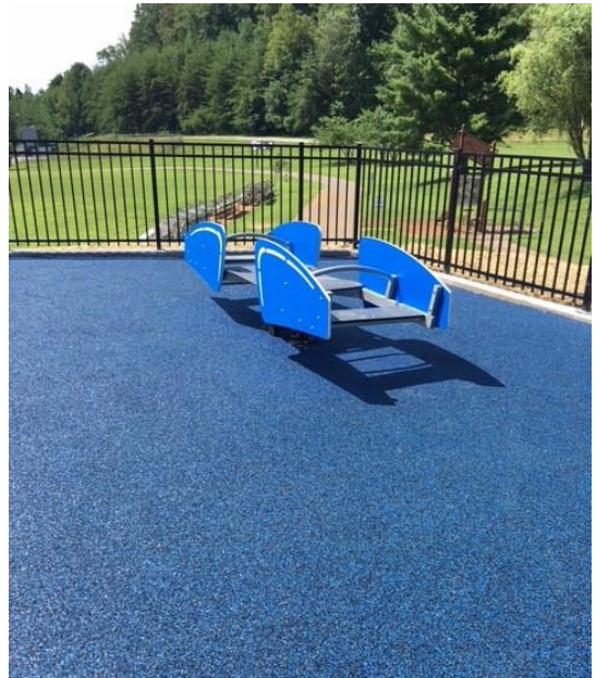
Photo 7: Poured-in-place rubber surfacing. Fischer Park, Somerset, Photo by Lisa Evans
