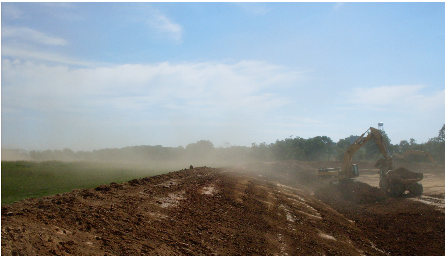
An example of fugitive dust emissions on a construction site. State regulation requires control measures such as spraying with water to reduce fugitive emissions and their impact on air quality. Photo: KY Department for Environmental Protection.
